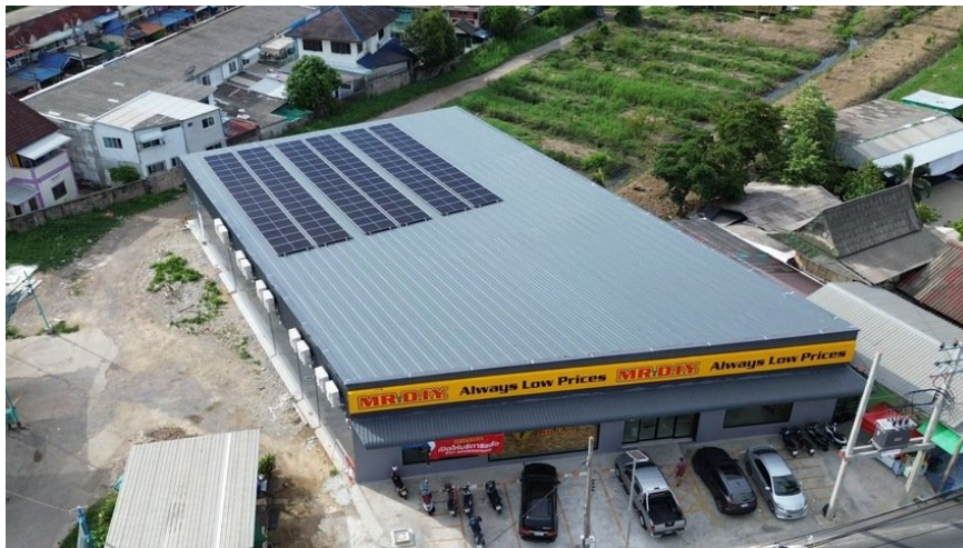
Solar Power Installation Project at Store
